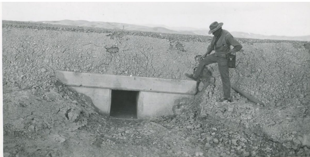
Figure 21. Built-up Fallon Sink grade and culvert, 1920. 153
